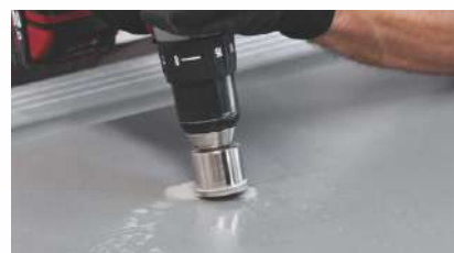
1. Round Cut with Diamond Blade Drill
