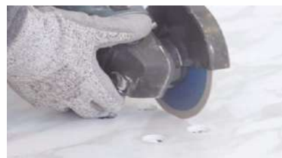
2. Cut with Diamond Blade Angle Grinder
