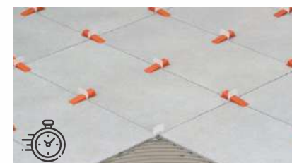
5. After Levelling Process leave it for 8-10 hrs.
