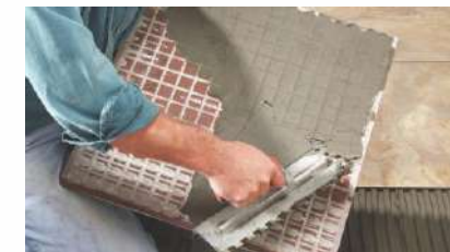
2. Cement laying on Tile
