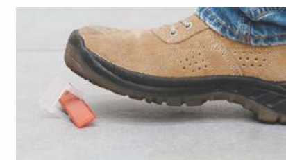
6. Remove Wedges ones it Dry
